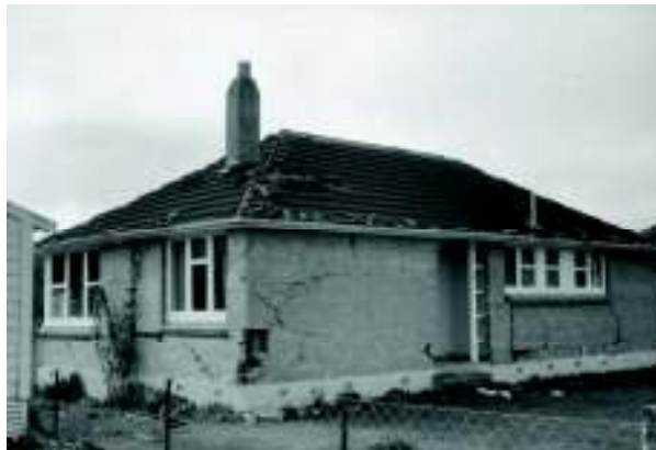
Inangahua earthquake, house damage, 1968 Barry Simpson, Nelson Photo news Collection 1226 fr6
