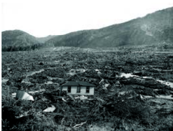
Busch's Slip and Morel's House, Murchison earthquake, 1929 NPM, F.N Jones Collection, 6x8 16
