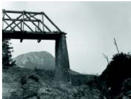
Murchison earthquake, 1929 (destroyed bridge) Kingsford Collection, 162198/5
